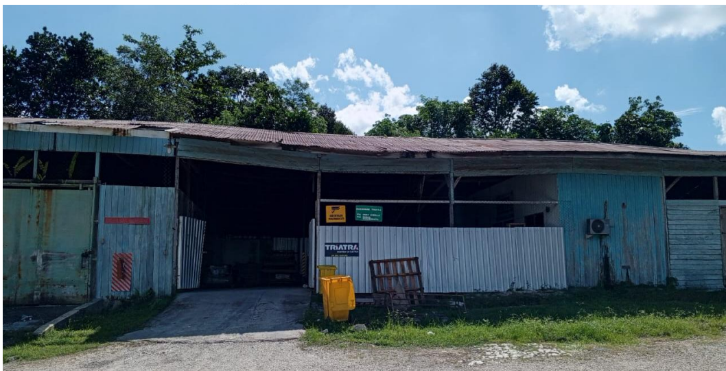
Gambar 3.1 Tampak Depan Warehouse PT. Triatra Sinergia Pratama Site Suaran
